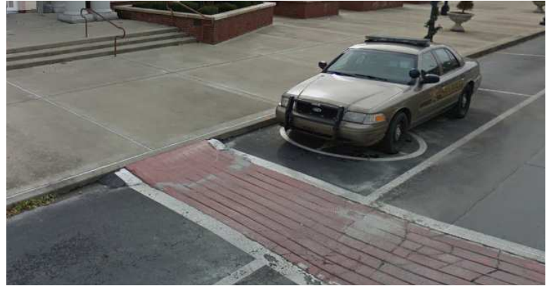
Example of ADA non-compliant midblock crossing on Main Street, lacking correct ramp and detectable warnings.
