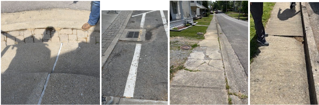
Several locations have older brick/stone pavers that have settled uneven and have created a tripping hazard. These uneven areas also have issues with water ponding and drainage. Other areas have cracked, or old or uneven sidewalk pavement.
