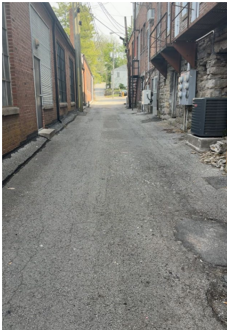
Several locations have older brick/stone pavers that have settled uneven and have created a tripping hazard. These uneven areas also have issues with water ponding and drainage. Other areas have cracked, or old or uneven sidewalk pavement.
