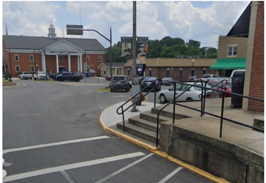
Example of ADA non-compliant intersection crossing on Main Street in Jamestown at Monument Square, lacking correct ramp and detectable warnings. Photo courtesy of Google.
