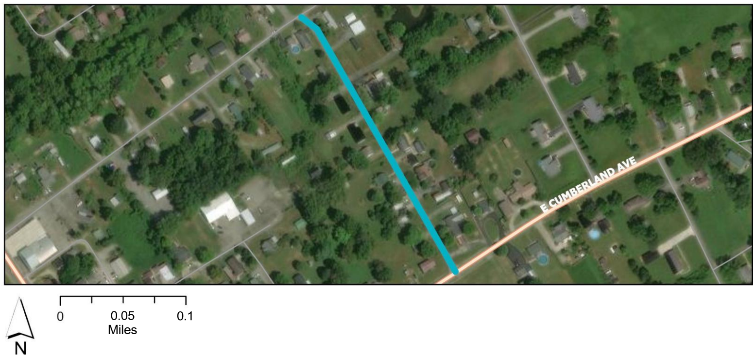
FIGURE 3.7 Popplewell Street Sidewalks in Jamestown
