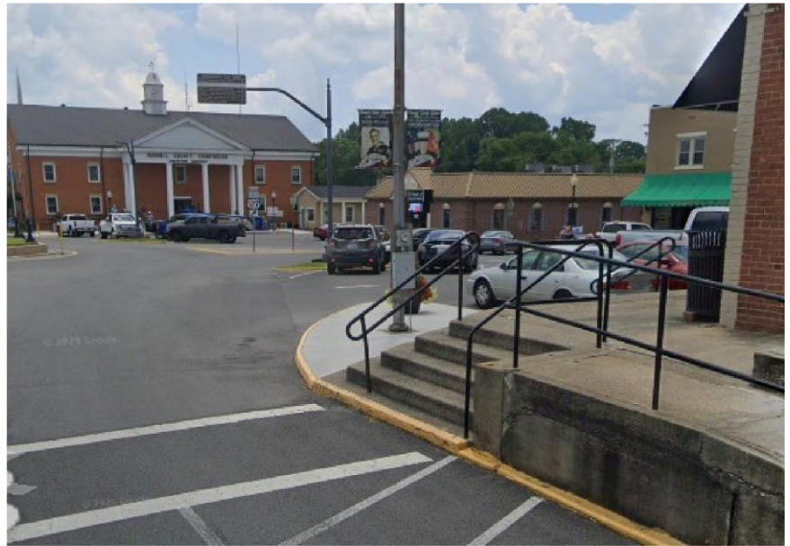
Example of ADA non-compliant intersection crossing on Main Street in
